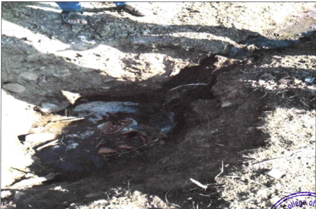
Shosh Khadda (Erosion Pit) Construction (17 th and 18 th January 2018)
